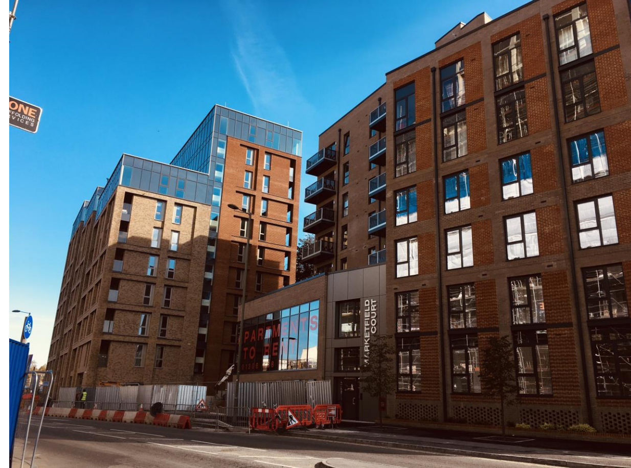
← looking at the building from in front of the site
